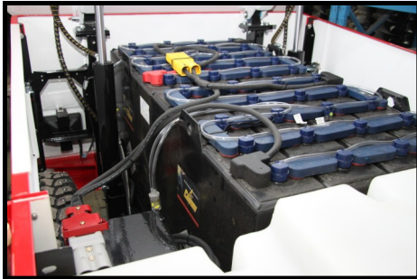
Batteries and cables ⇒ Batteries 552
